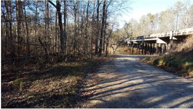
PHOTO 8 ENOREE RIVER BRIDGE INFORMAL ACCESS AREA
