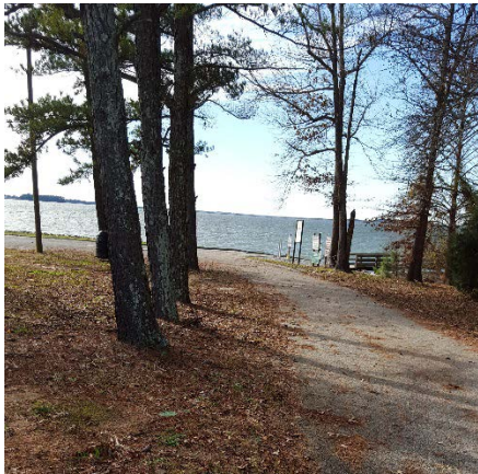
PHOTO 2 HIGHWAY 215 BOAT RAMP
